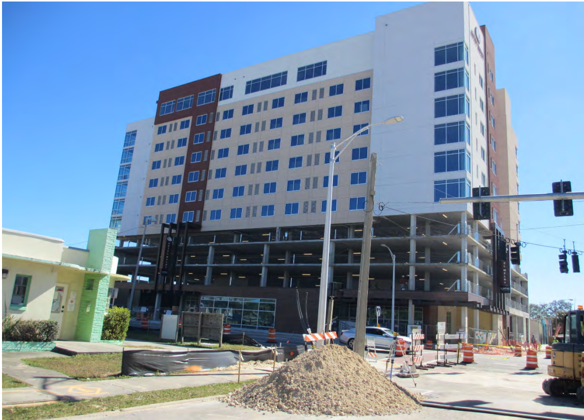
FIGURE 3 - HILTON TAPESTRY/HOTEL MELBY RENDERING & UNDER CONSTRUCTION
