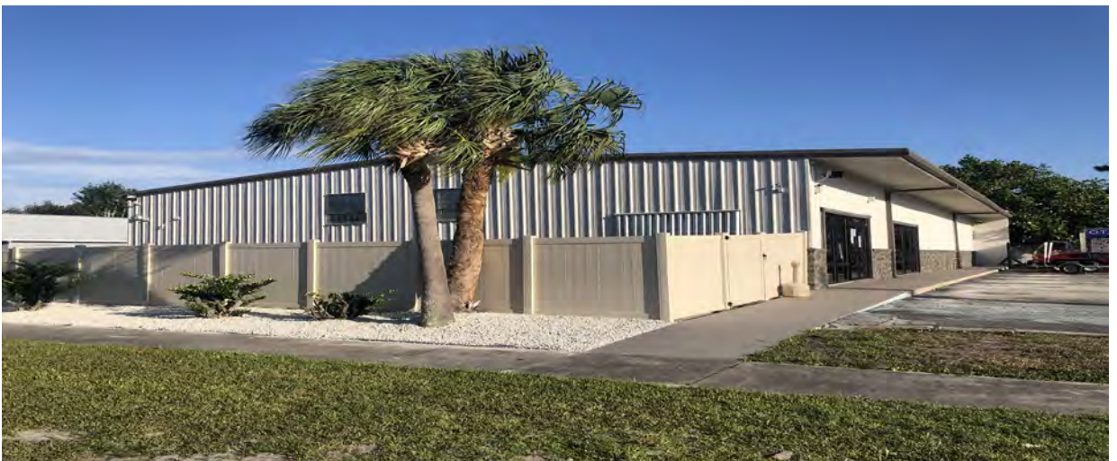
FIGURE 4 – 201 S. BABCOCK STREET FACADE IMPROVEMENT BEFORE & AFTER FRONT & SIDE ELEVATIONS
