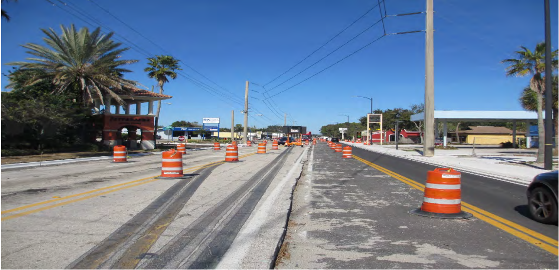
FIGURE 5 - BABCOCK STREET PHASE III-B MEDIANS – UNDER CONSTRUCTION
