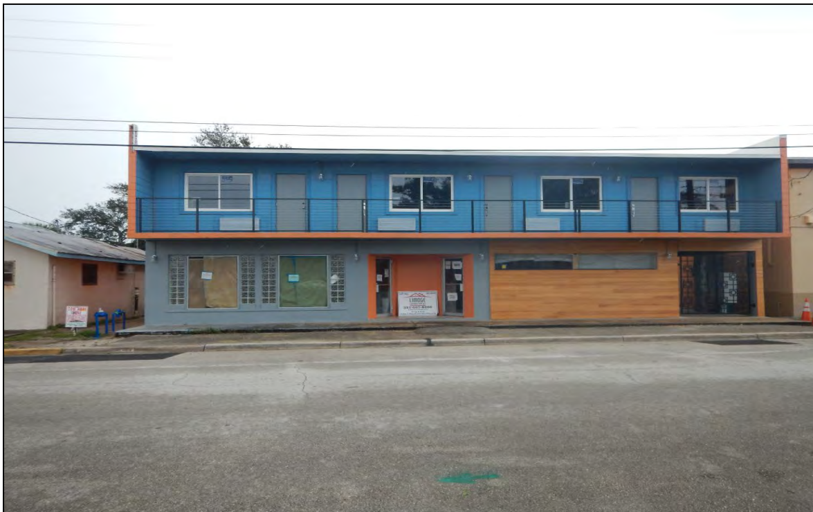
FIGURE 1 – 2421 STONE STREET FAÇADE PROJECT - BEFORE & AFTER
