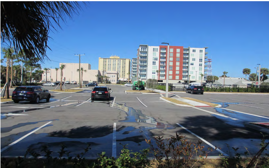
FIGURE 2 – HIGHLINE COMPLETED CONSTRUCTION AND PUBLIC PARKING FACILITIES
