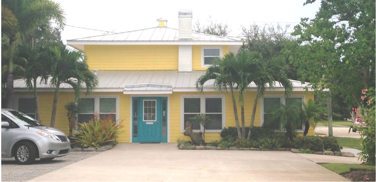
Figure 8: Main (South) Façade
