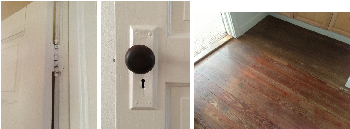
Figure 12: Original Interior Features (Second Floor)
