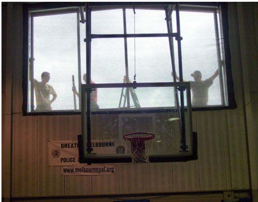
REPLACEMENT WINDOW IN GYMNASIUM GRANT ST. C.C.
