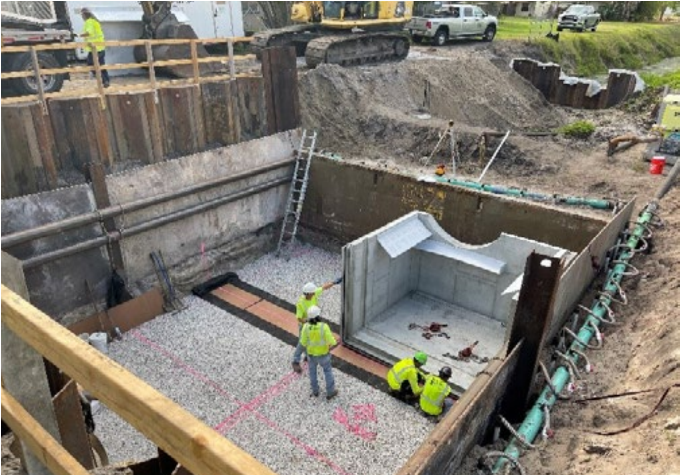
Thrush Drive Baffle Box under construction.
