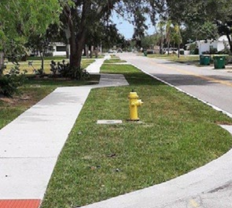
New sidewalks were constructed.
