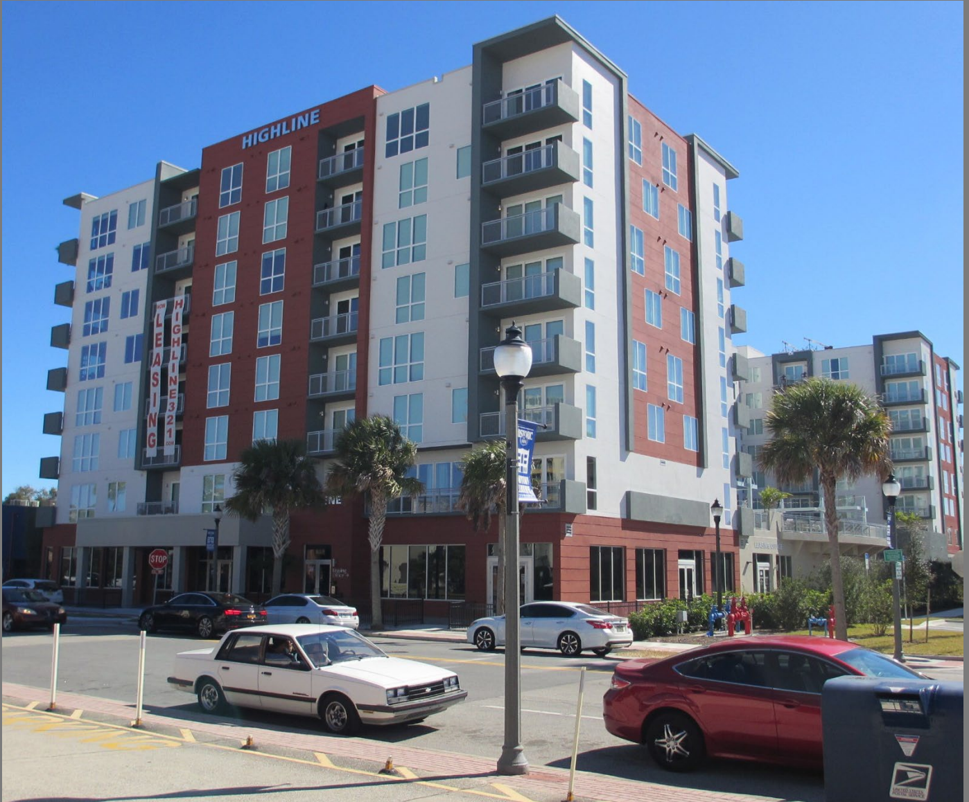
PICTURED ABOVE IS THE COMPLETED HIGHLINE APARTMENT PROJECT
