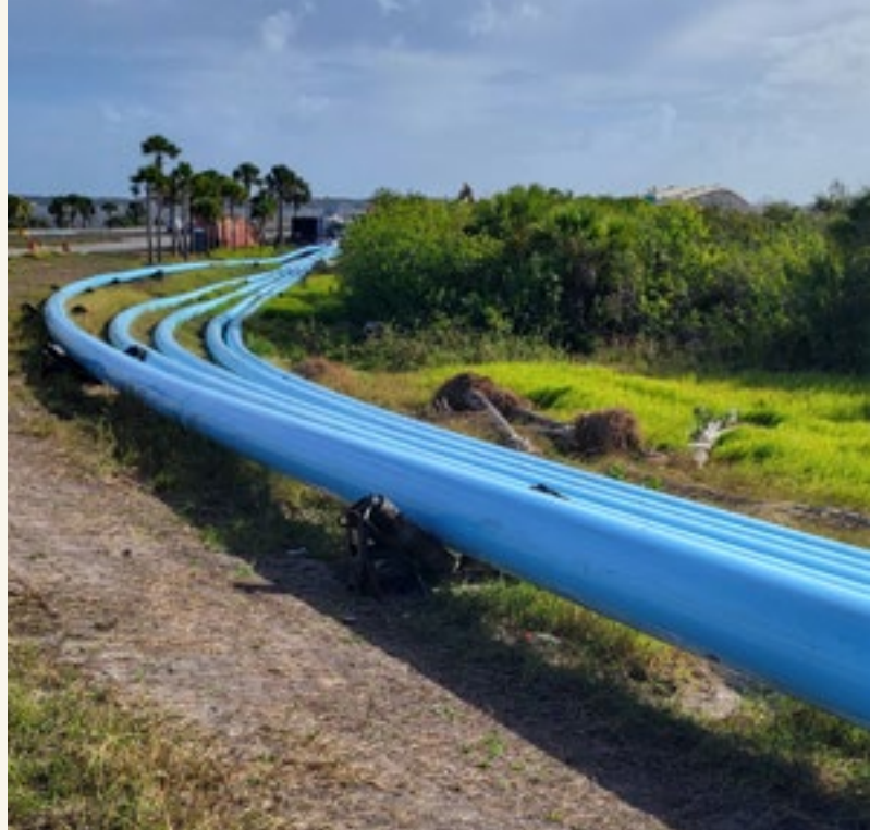
Fusable pipe ready for directional drilling along Pineda Causeway.
