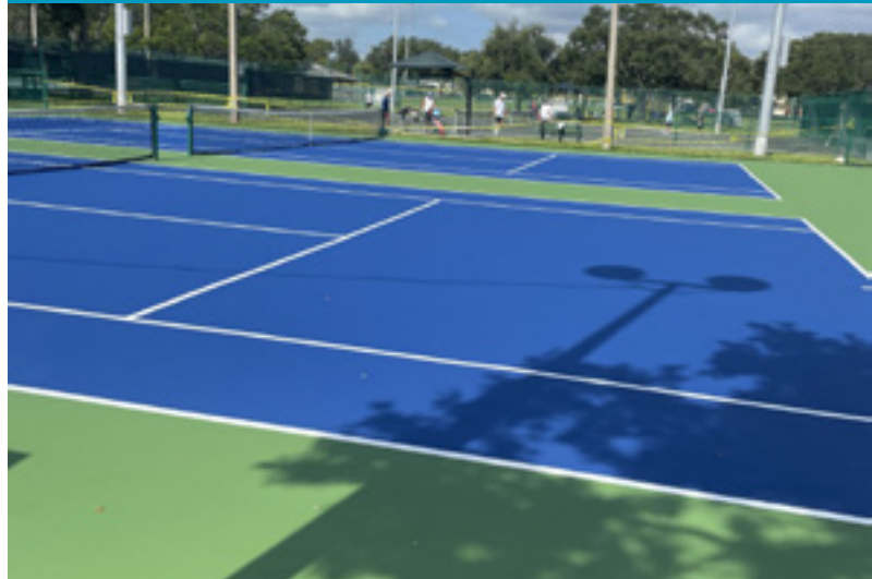
Resurfaced Tennis Courts at Fee Avenue
